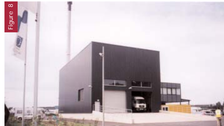
Figure 8 shows an RDF plant (using Energos technology) in Germany that is handling roughly the same amount of RDF as the plants we will need, namely 40,000 tonnes per year.
